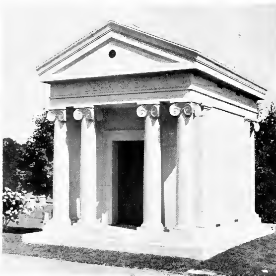
Number 8793. Ionic style of architecture unusually strong of construction. The interior is of marble finish with a polished granite floor. Erected for Mr. Wm.M.Knox, in Oak Park Cemetery, New Castle, Pa.
